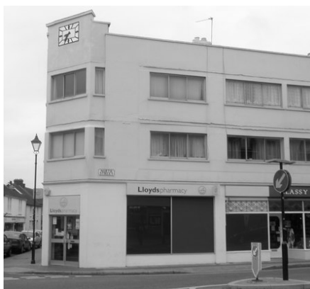
Central Buildings on the corner of West Street
